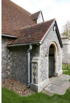
A number of put-log holes, used for the erection of wooden scaffolding during construction of the building, can be seen on the walls of the Lady Chapel and the tower.
